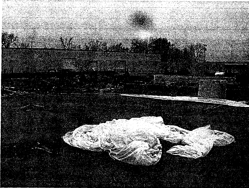
Date: February 24, 2005 Time: 12:14 pm Direction: SW Photo by: M. Cozadd Exposure #: 009 Comments: Overview of debris near northeast corner of site.
