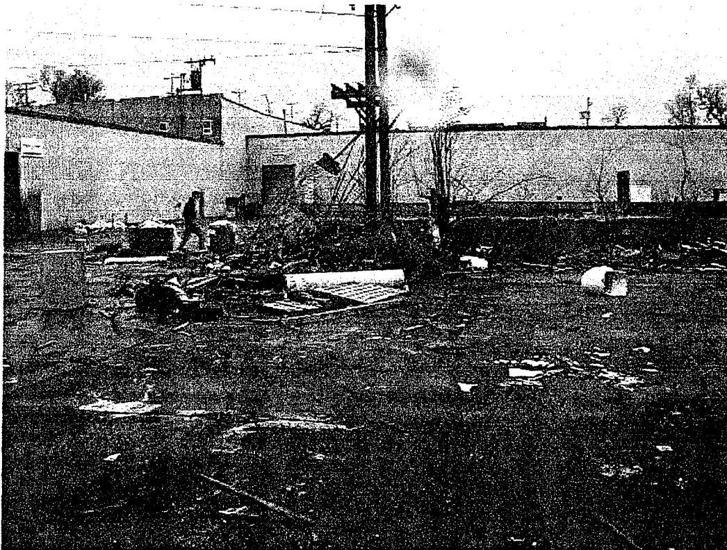
Date: February 24, 2005 Time: 12:14 pm Direction: S Photo by: M. Cozadd Exposure #: 010 Comments: Overview of debris near northeast corner of site.
